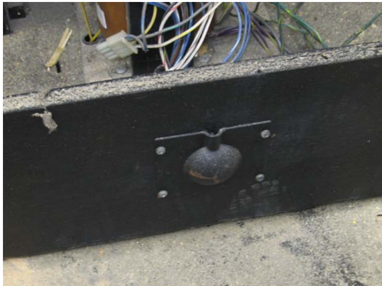
Figure 25 - AC Line Cord Relief Plate
