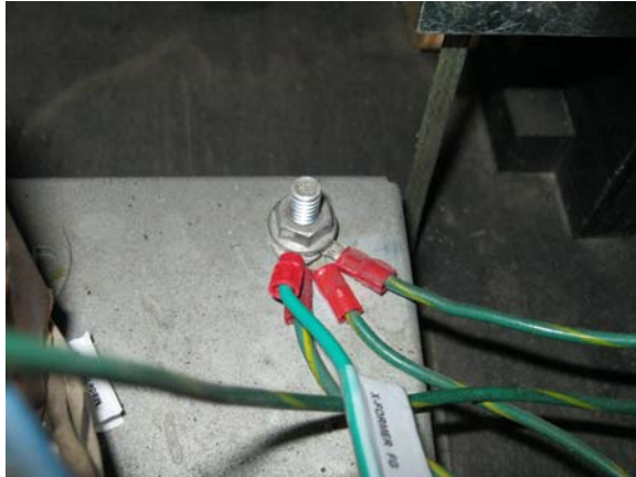
Figure 49 - Transformer Chassis Plate Grounds
