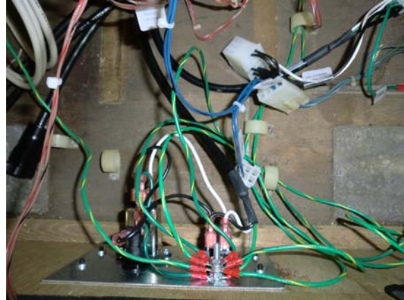
Figure 50 - AC Power Plate Grounds
