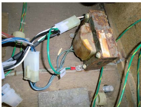
Figure 47 - Exotica Transformer Connections
