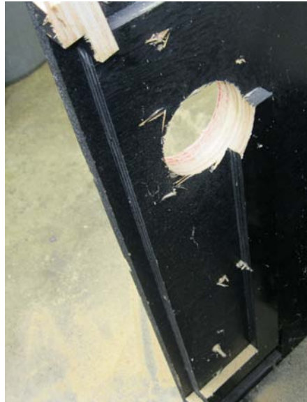
Figure 23 - Cleats and Strips Need to be Removed
